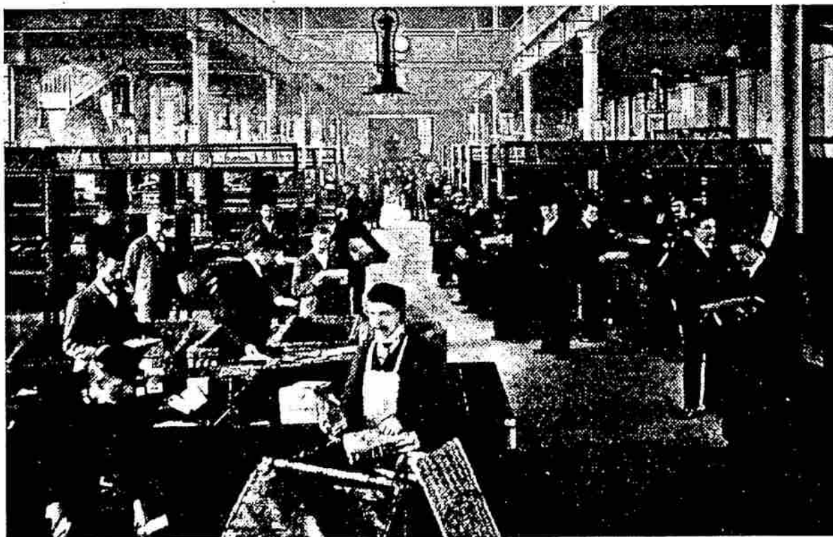
Parcel Post Sorting Room. New Bridge St. Strangeways 1894
